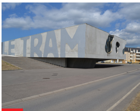
Centre culturel TRAM, avenue Marguerite Duras.
